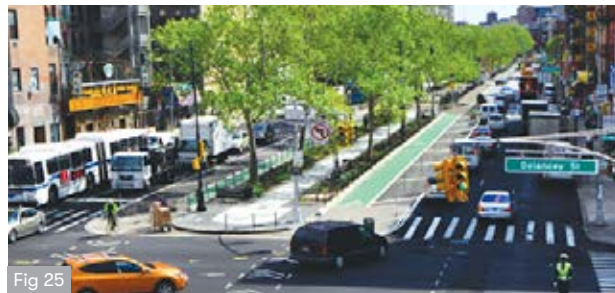
Fig 25 Allen Street, NYC was transformed with a pedestrian promenade and dedicated bike lanes
